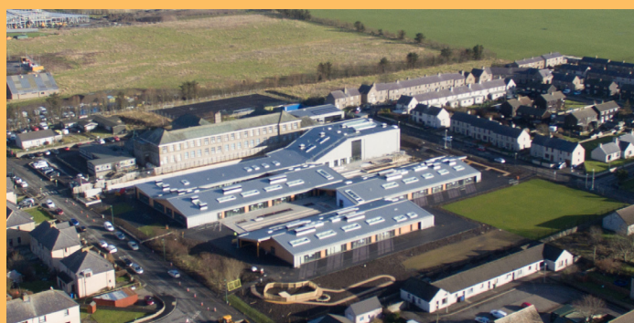
A bird's eye view of the new Noss Primary School in Wick.
