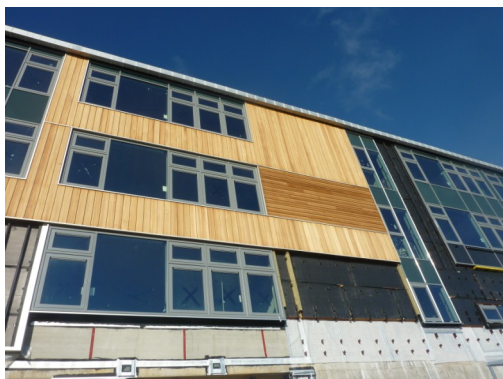
Cladding on South side of school
